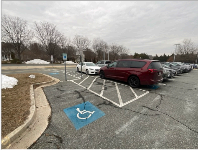
OVERVIEW OF ACCESSIBLE PARKING AREA
