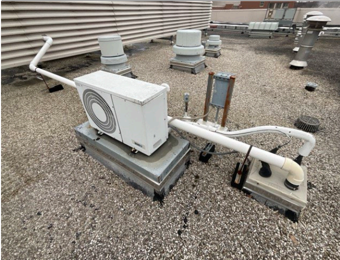
7 - SPLIT SYSTEM DUCTLESS
