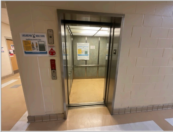
LOBBY LOOKING AT CABS
